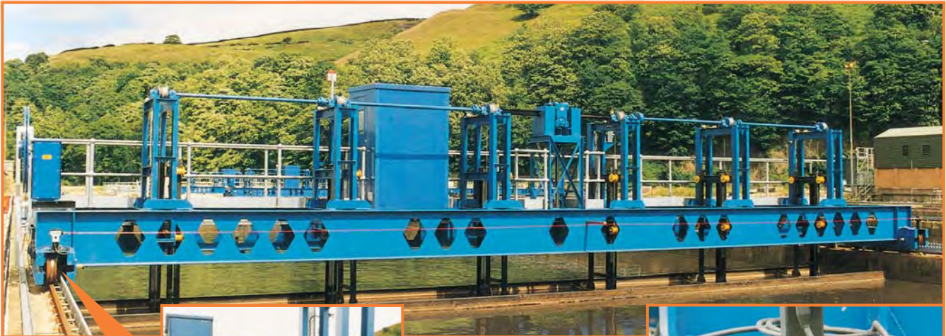
Bridge scraper for rectangular settlement tank
