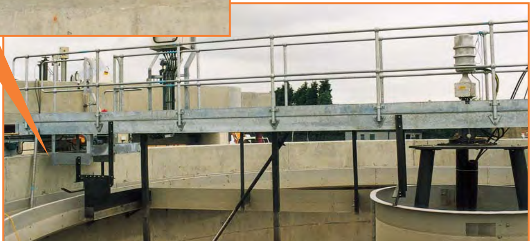
Half Bridge scraper for rotary settlement tank
